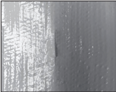
1. Locate the damaged area
